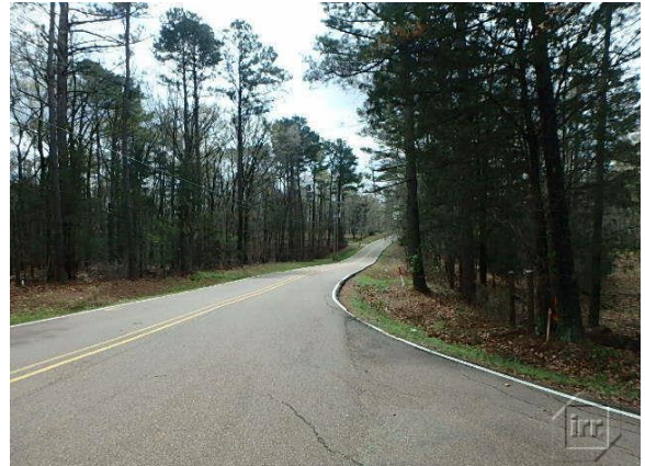
View of Lake Cavalier Road (Photo Taken on March 13, 2016)
